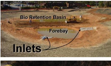
Forebays cost less to construct than a sump and SAFL Baffle but the annual costs to maintain each is significantly higher for forebays.
