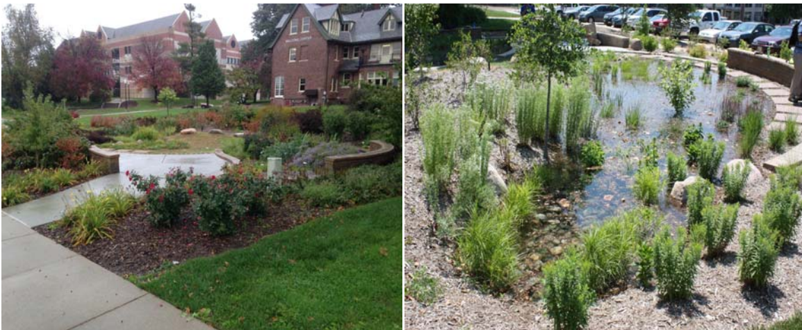
Figure 4. Photographs of the bioretention systems in front of the UNO Welcome Center (left) and the North bioretention system entirely inundated (right).
