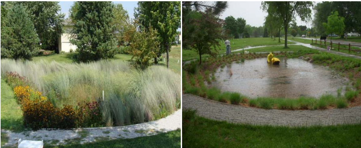
Figure 5. Photographs of the bioretention system at Orchard Park exhibiting vigorous summer growth (left) and fully inundated during a rain event (right).
