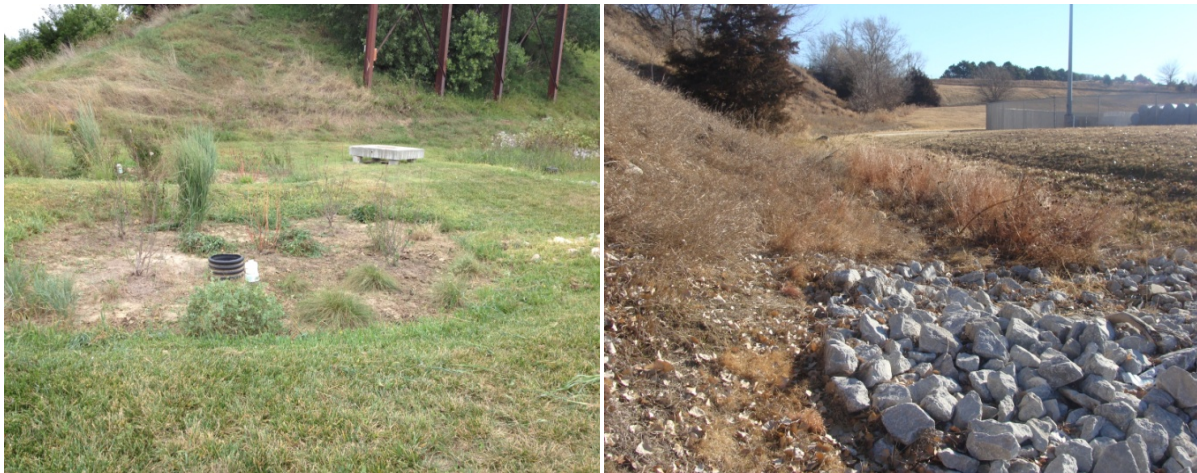
Figure 8. Photographs of the bioretention systems at the Under the Sink facility (left) and the bioswale that drains in bioretention system 1 (right).
