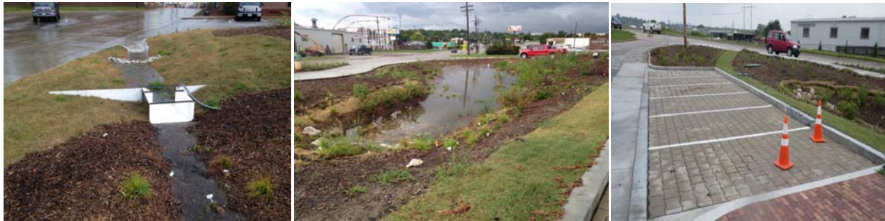
Figure 12. Bioretention system at Sewer Maintenance Facility partially inundated after a rain event (center), with West forebay (left), and permeable paver parking lot (right).
